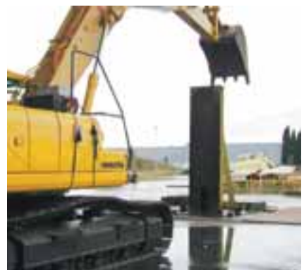
PC340 demolition machine, twisting load applied to new demolition first boom.
