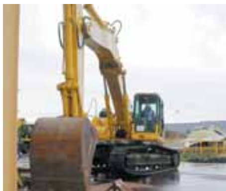
PC340 demolition machine, digging boom installed, with simultaneous twist and bend loading.
